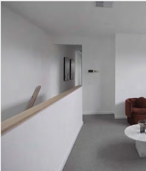
Stained timber capping
