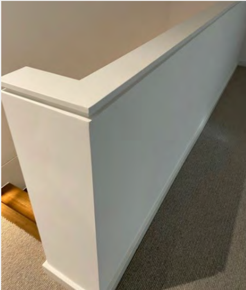
Plaster lined dwarf wall with painted MDF capping to top of stair
